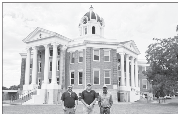
Photo provided Local roofers Greg Newman Sr., Gregory Newman and Keeton Manuel stand in front of the Love County Courthouse after completing its new roofing project.
