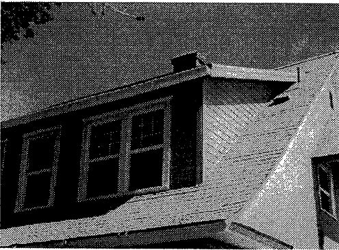
Dormers should be placed in from the eaveline of the house, as these original dormers illustrate.
