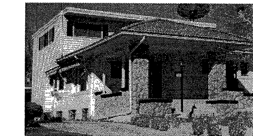
A second story addition that follows the pitch and roofline of the main part of the house, and is set back from the plane of the front wall, will go a long way from detracting from the historic appearance of a house (above). Additions like this are incompatible with the massing and form of the original house, and should not be constructed (below).
