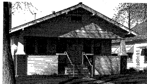
An intact example of a typical porch on a Craftsman bungalow.
