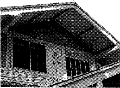
The storm window on the dormer of this house is flush with the wall, is compatible in color to the other windows, and does not compete with the pattern of the window itself.
