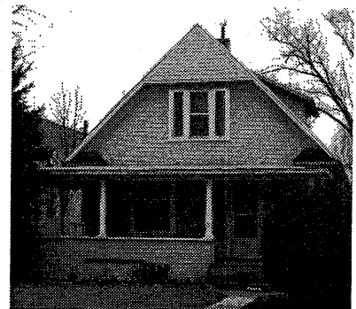
Examples of Transitional Colonial Revival. Like the four-square, this style is far outnumbered by the bungalow in older Twin Falls neighborhoods, but their presence contributes to the rich architectural legacy of this young community.
