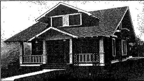
The Henry and Jessie Failing house on Tenth Avenue N., constructed about 1910. Failing was a bank vice-president. It has changed little over the decades.
