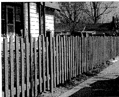
All the fences illustrated here have a transparent quality, and are in character with the architecture of older neighborhoods. Wood picket fences are a popular fence type, and appropriate for all styles in the city's neighborhoods except the Prairie style. This fence (center) has a unique design, but the use of wood material makes it compatible with the historic character of the streetscape, and the use of lattice keeps it from being imposing to passers-by. Wrought iron is an alternative material because it was used historically and can be seen through.
