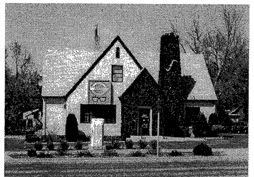
In 1936 the subsequent owner, John E. Hayes, transformed the McCollum house. Because the changes occurred over fifty years ago (the period preservationists consider a minimum for structures or alterations to achieve historic significance) a property owner should consider alterations that respect its Tudor Revival character, of which it is a good example. (Tudor Revival styles are described on page 12).
