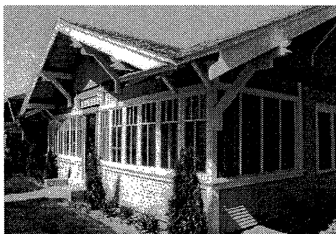
The scale and design of the windows of this enclosed porch make it compatible with the design of this Craftsman bungalow.
