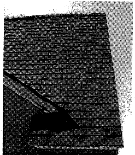
The pattern and profile of these shingles of this asphalt roof are appropriate to the style of this Tudor Revival style house (above).
