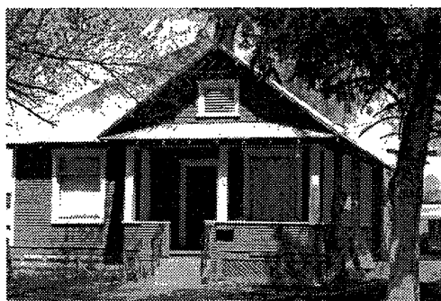
This dwelling has little ornamentation. It achieves its style through its massing, the shape and design of its windows, the exposed rafters, the design of the porch and the concrete block foundation.
