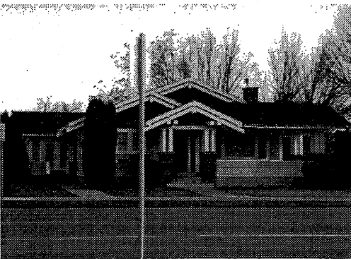
An example of an "airplane" bungalow, so categorized because its strong horizontal lines resemble the wings of an airplane, and because the placement of the highest gable imitates a cockpit. Robert McCollum moved from his Victorian-style home illustrated on the previous page to this residence about 1914.
