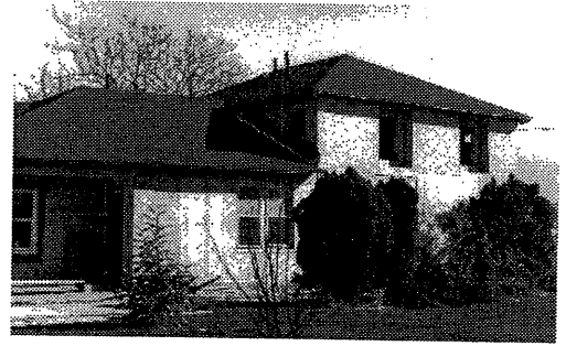
Although the addition in this example is unfinished, the massing of second story addition follows that of this modest house. The addition will be subordinate because it is set back from the front of the house.
