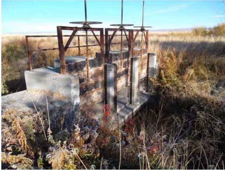
Concrete headgate structure at Little Wood River diversion
