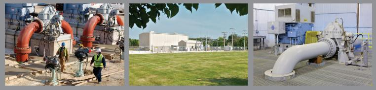
Open air and enclosed pump station units are designed to increase the pressure in the pipeline in order to maintain flow to keep the liquid petroleum moving at about walking speed.
