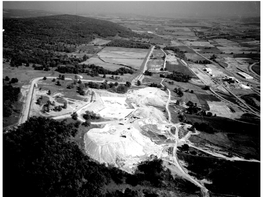
Figure 5: The reservoir construction site with the concrete sides poured, looking east. The Baraboo Hills slope up to the left. The massive spoil piles are downslope of the reservoirs. The buildings in the upper right are part of the TNT Acid area.
