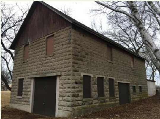
Above: Park shelter and stone barn.
