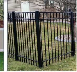
No Dig fence installations drive posts deep into the ground with metal posts hidden. The end result is a stronger, longer lasting fence with no dirt mess behind from digging holes.
