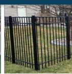
No Dig fence installations drive posts deep into the ground with metal posts hidden. The end result is a stronger, longer lasting fence with no dirt mess behind from digging holes.
