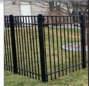
No Dig fence installations drive posts deep into the ground with metal posts hidden. The end result is a stronger, longer lasting fence with no dirt mess behind from digging holes.
