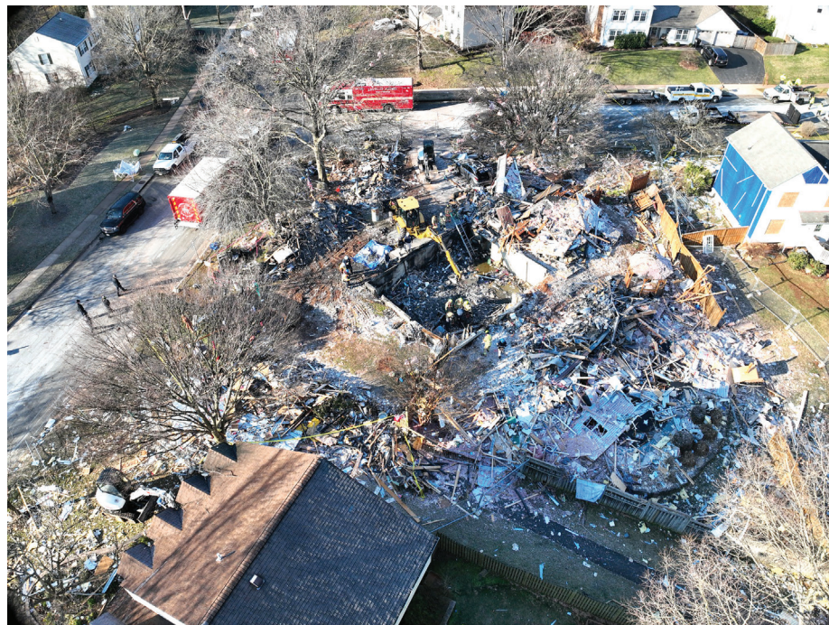
An overhead view shows the damage after a home exploded in Sterling Feb. 16, after an unknown ignition source sparked leaking propane.
