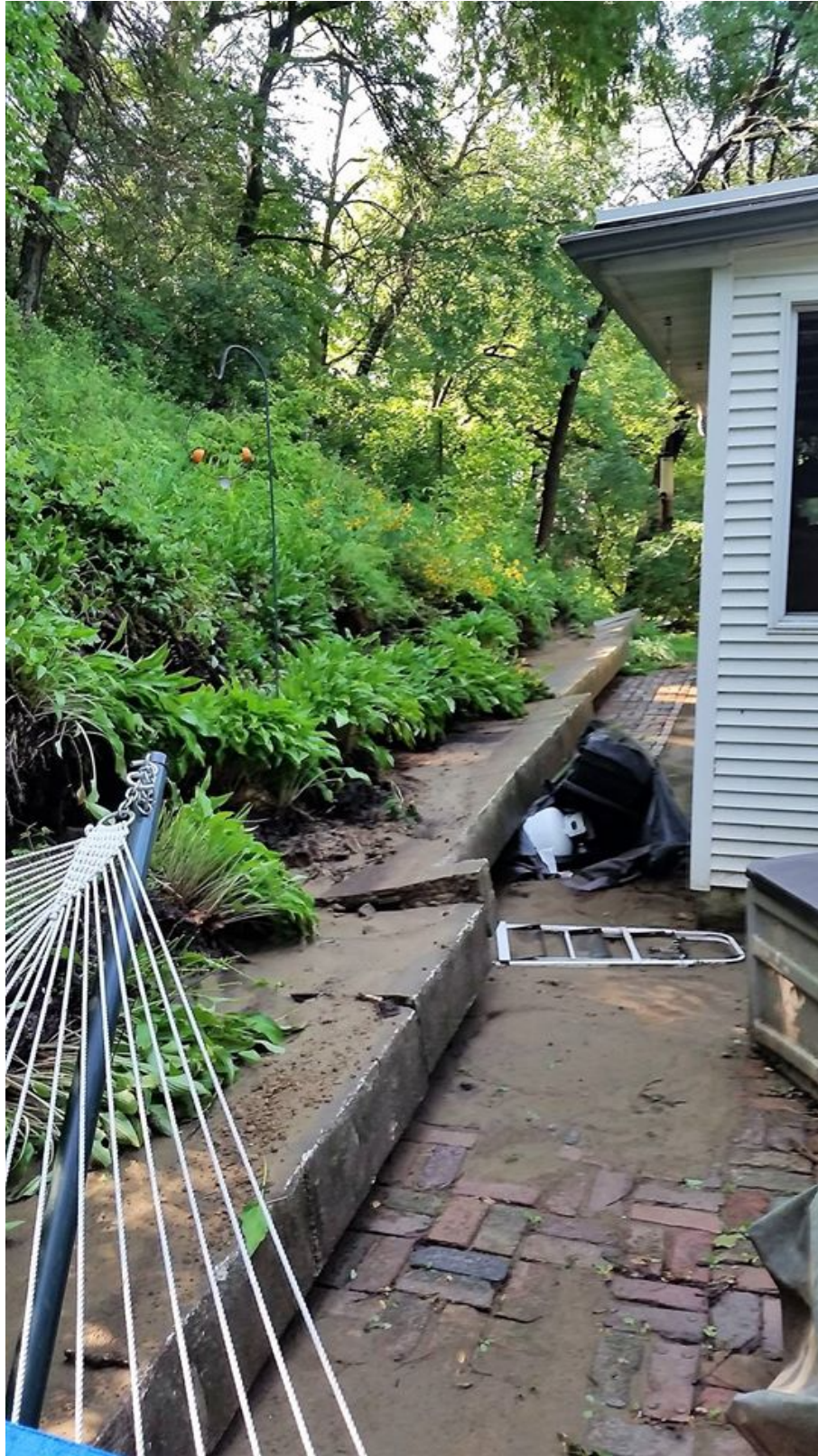
Figure 4. Evidence of bluff instability as manifested by retaining wall failure.
