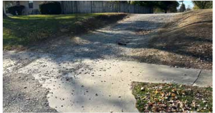
Entrance at Mendota Park - Steep entrance with gravel.
