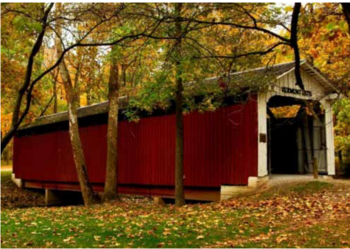
Vermont Covered Bridge Image Source: www.visitkokomo.org
