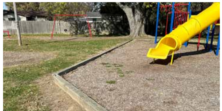
Playground surfacing and edging at Mohawk Park - Mulch is not considered an accessible safety surfacing, the edging is not flush with ground and there is no accessible path to the amenity.
