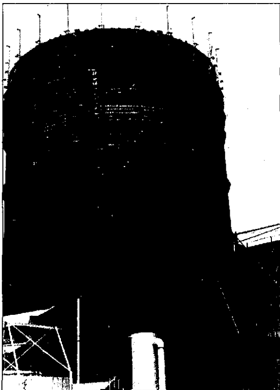
ALMOST THERE: In this photo, the work is being done on the fifth gallery of five total. Completion of the elevator shaft and stairway takes place during this phase.
