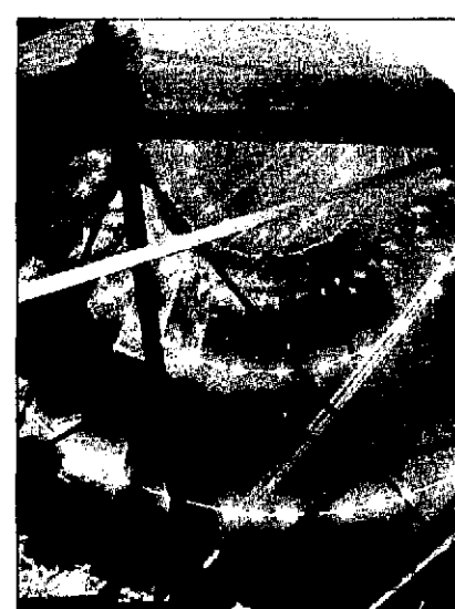
LOOKING UP: Light streams in from holes cut in the top of the tower in preparation for the demolition.
