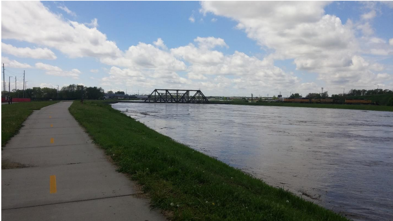
Figure 8. Salt Creek Flood Risk Reduction Project.
