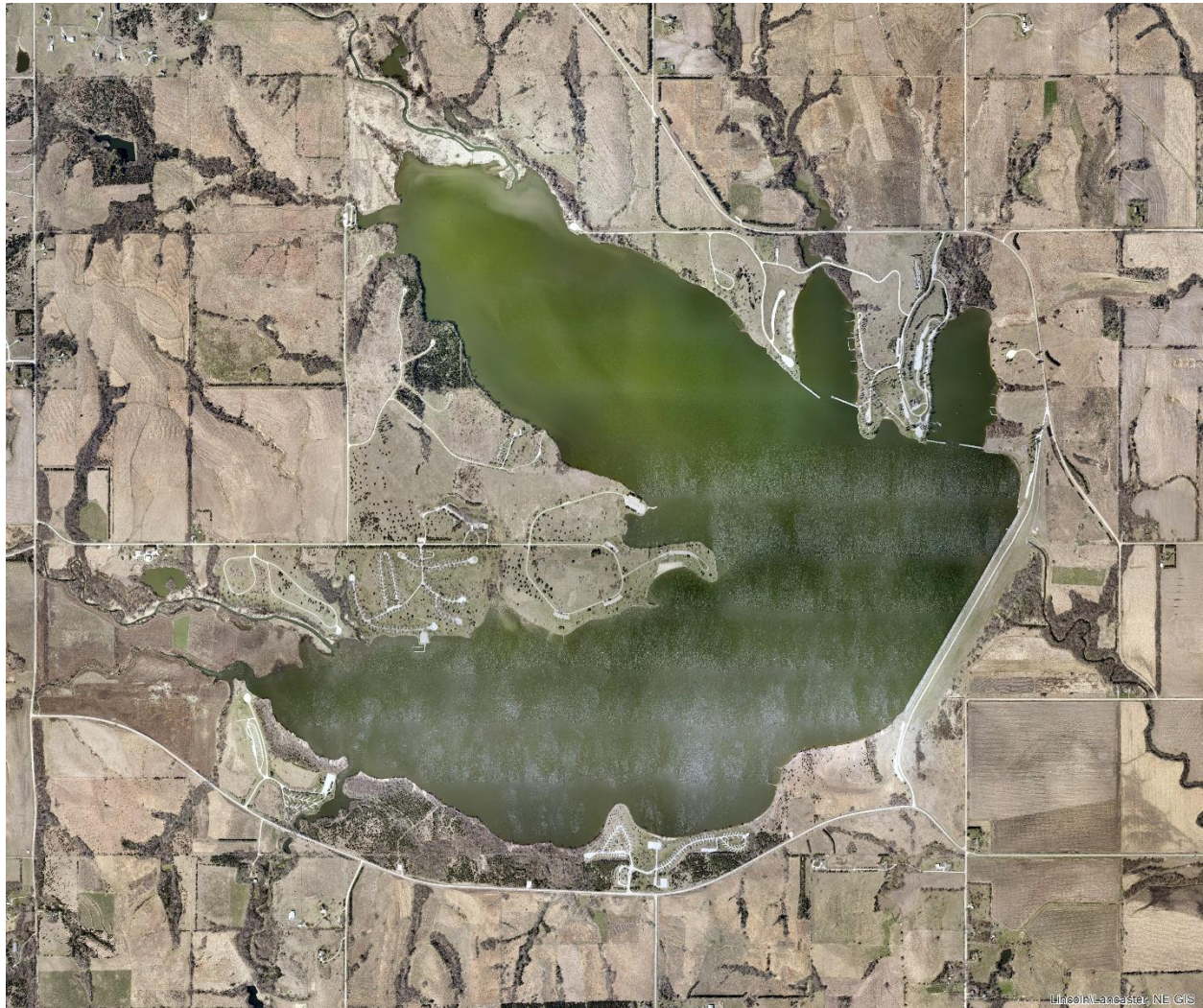
Figure 7. Branched Oak Lake – One of 10 Large Flood Management Dams Built by the U.S. Army Corps of Engineers (USACE).
