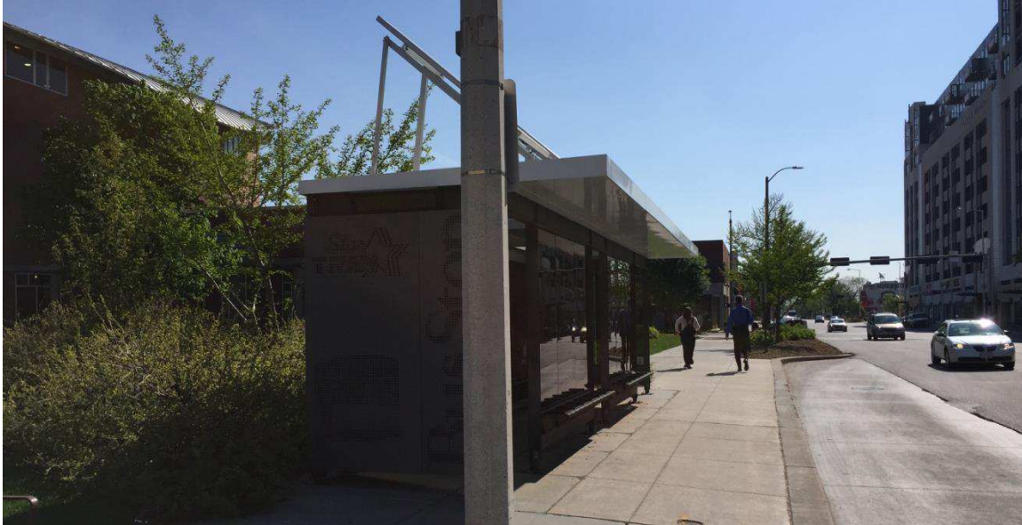
Figure 111 StarTran Downtown Bus Stop Shelter
