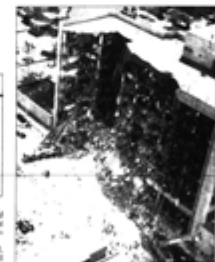
The federal building in downtown Oklahoma City sits in ruins after Wednesday's bomb blast. At least 12 of the dead were children.
