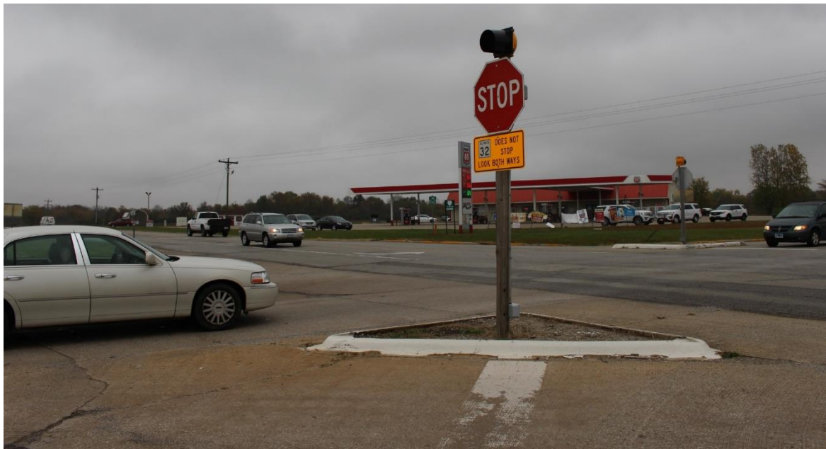
Figure 19 - EXAMPLE OF DETERIORATING PAVEMENT MARKINGS AND NO STOP BAR PRESENT
