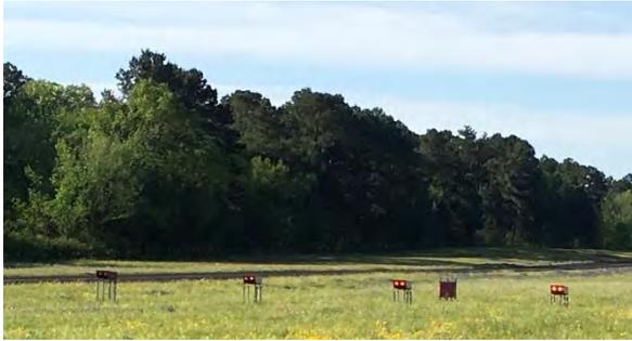
Each runway end, outboard of the threshold lights, is equipped with light emitting diodes (LED) REIL.
