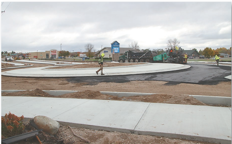
The first layer of asphalt for the Isanti roundabout was being put into place on Wednesday, Oct. 22. Work is scheduled to be completed by the end of October.
