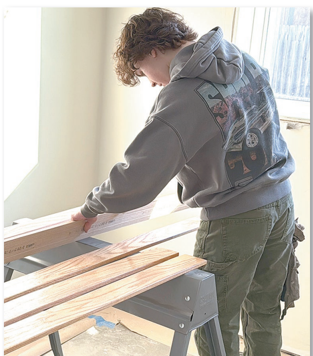
CONTRIBUTED A student from Pine Technical College’s construction technology group stains baseboards before installation.
