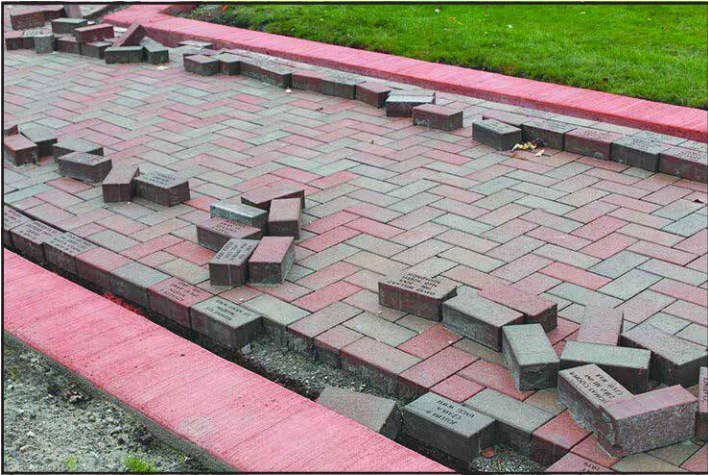
Photo by Kaitlyn Campbell RE-INSTALLING BRICKS – The brick pavers at Tawas City Veteran’s Park are usually set into their slots, but right now, many are pulled up and the path entryways are lined with yellow caution tape. This is because new curbing has been installed to keep them in place, which will require a re-laying of all of the existing bricks.
