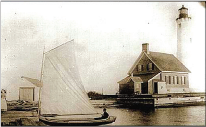
When erected in 1876, the Tawas Point Lighthouse rested on a timber crib and was completely surrounded by water. By 1891, accretion (the movement of sand by wind and water) resulted in the lighthouse being completely surrounded by land.
