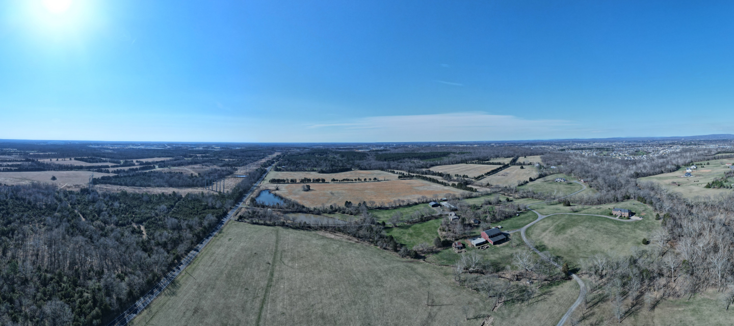
Manassas Battlefield Historic District (Nat'l Register of Historic Places) facing complete destruction from the PW Digital Gateway
