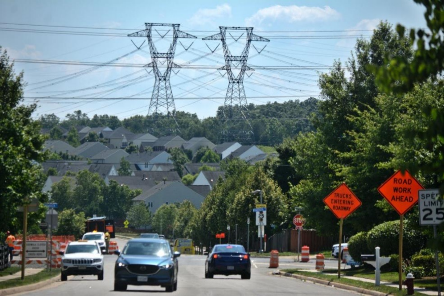
Power lines over homes in Kirkpatrick Farms, viewed from Supreme Drive in Aldie,VA
