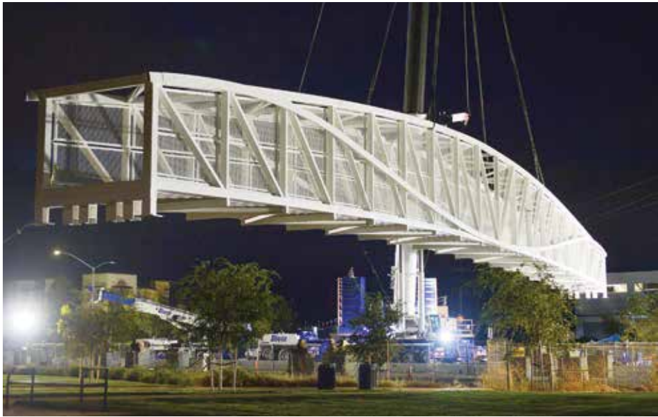
The Iron Horse Trail/Dublin Boulevard Overcrossing bridge was placed in position during the early hours of Sunday, Oct. 22. The free-span bridge will provide a safe crossing for trail users and facilitate improved traffic flow. The main structure is approximately 230 ft. long and 20 ft. high. (See photo gallery at www.independentnews.com/multimedia ) (Photo – Doug Jorgensen)
