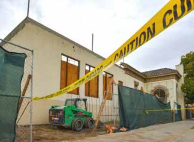
The former SBC Building at 2324 Second St. in downtown Livermore remains under renovation, delaying the opening of the Farmers Union restaurant by more than a year. The building was constructed in 1928 as the city’s first purpose-built telephone exchange. (Photo — Doug Jorgensen)
