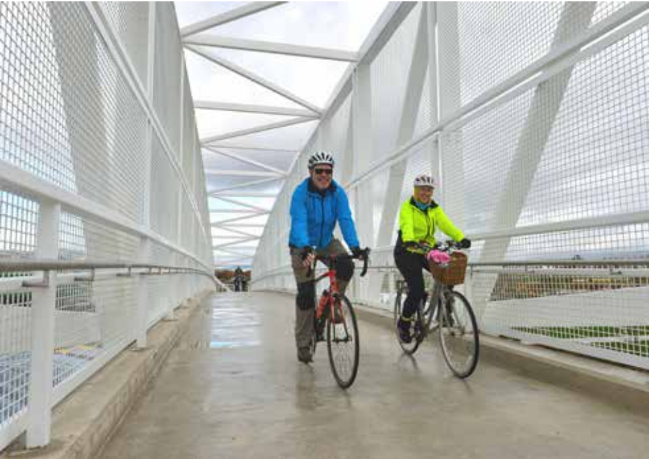
Walkers and riders enjoyed their first opportunity to cross the new Iron Horse Trail bridge, which curves above busy Dublin Boulevard near Don Biddle Community Park. (Photo — Doug Jorgensen)
