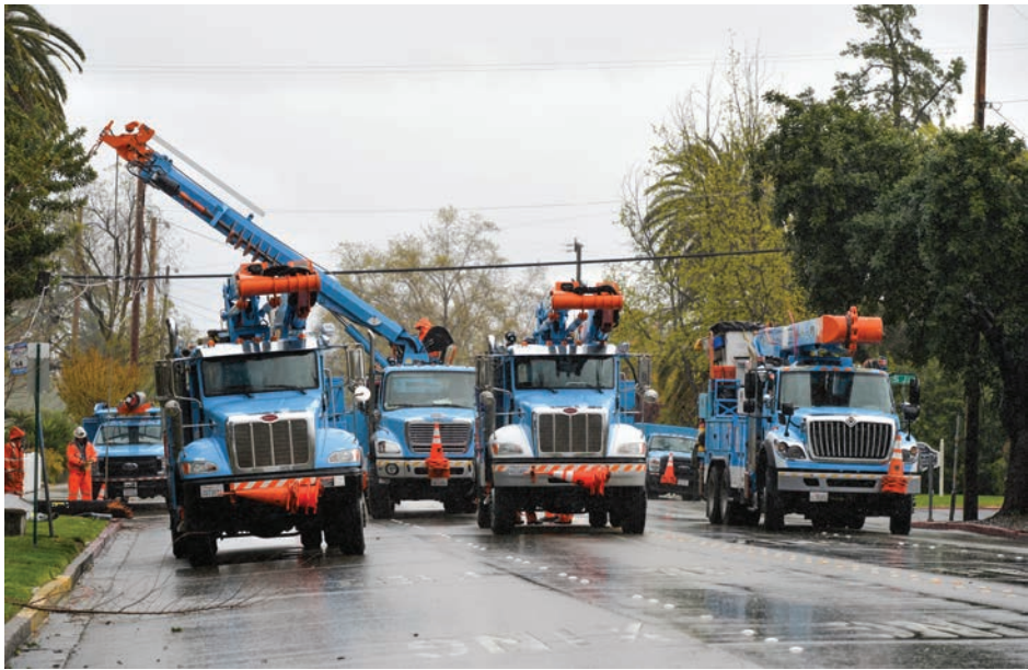
PG&E closed a portion of 4th Street near Carnegie Park in Livermore to replace a damaged power pole on Sunday morning, April 5. (Photo - Doug Jorgensen)
