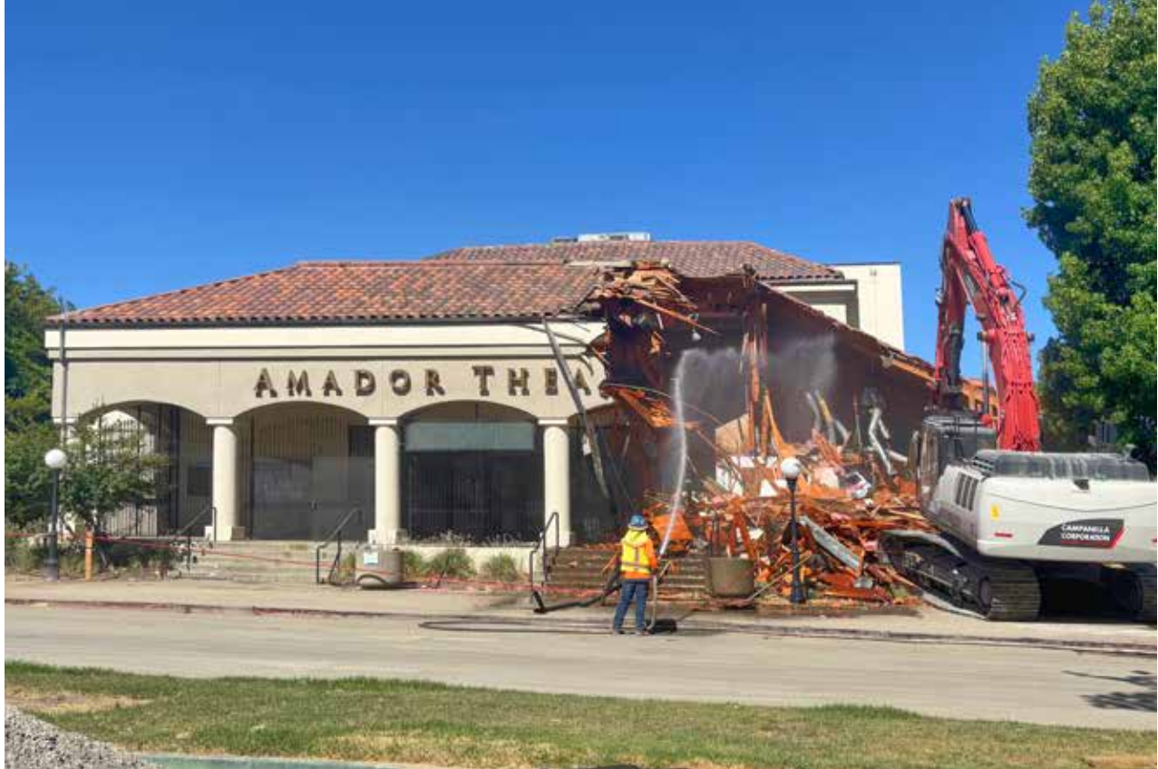
Heavy machinery begins the demolition of Amador Valley High School’s longtime theater, clearing space for a modernized, multi-purpose performing arts center scheduled to open in late 2028. (Photo courtesy of PUSD)
