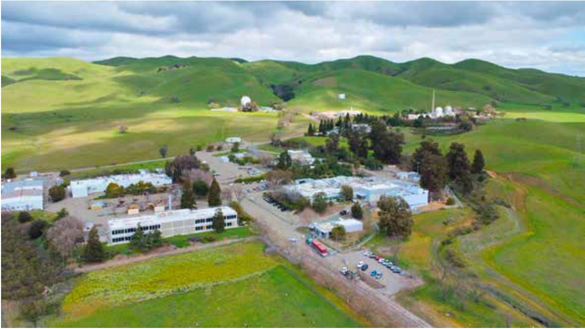
This aerial photograph captures the 1,600-acre Vallecitos Nuclear Center, nestled in the rolling hills near Sunol. The wide view shows the complex of buildings and infrastructure that Zeno Power intends to revitalize for its new manufacturing facility. Existing research buildings and laboratories sit among open fields, adjacent to a section of larger structures, some dating back to the site's historic operation as the nation's first privately owned nuclear plant. NorthStar Group Services continues decontamination and decommissioning efforts across the broader site. (Photo courtesy of Zeno Power)
