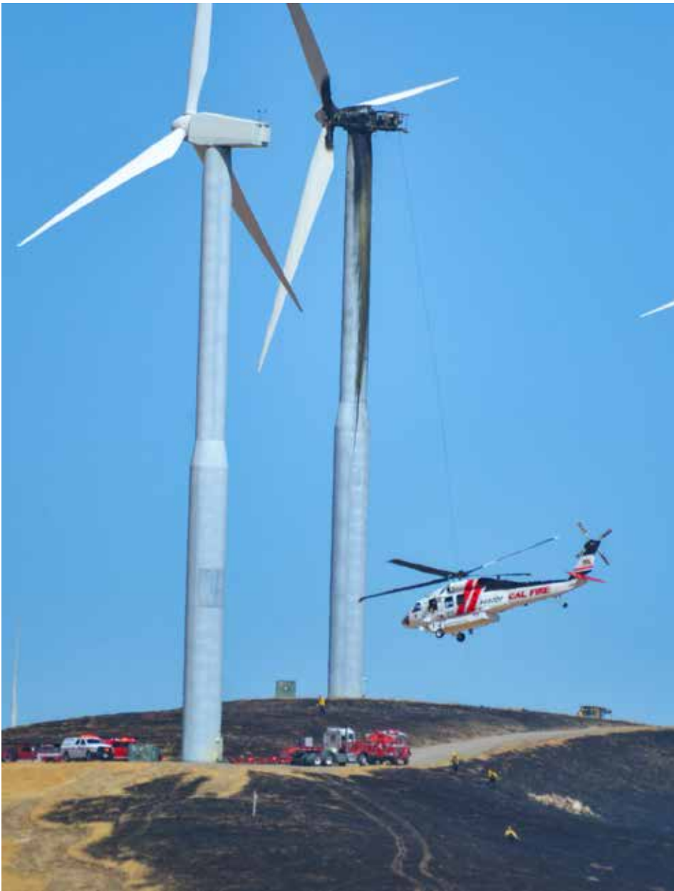
Cal Fire crews work an incident involving a burning wind turbine on June 26. Located near the intersection of Altamont Pass Road and Grant Line Road, the blaze grew to 20 acres before firefighters contained it on the afternoon of June 26. (Photo – Doug Jorgensen)
