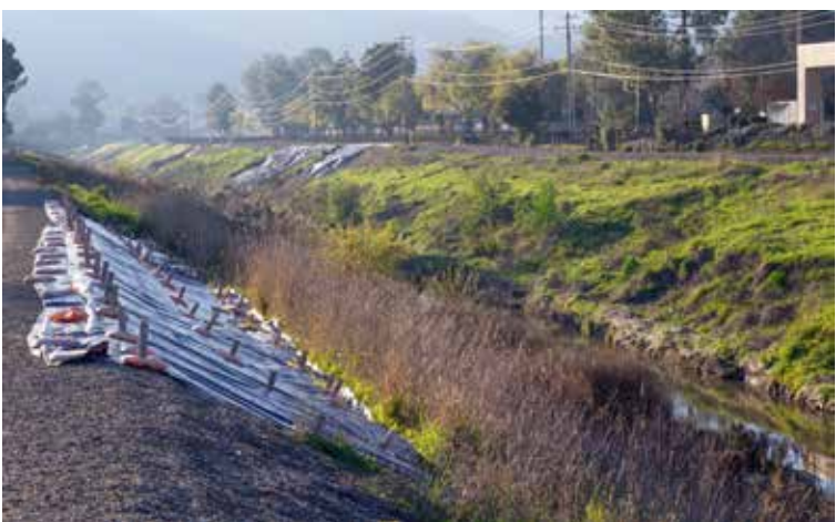
Temporary repairs help stabilize the bank of the Arroyo Mocho near Hopyard Road in Pleasanton. Zone 7, the City of Pleasanton and the U.S. Army Corps of Engineers repaired stream banks and enhanced flood protection in the area last fall. (Photo — David Jen)
