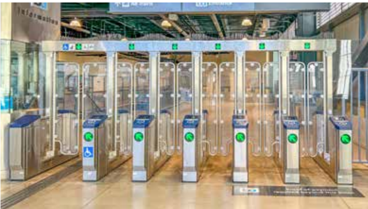
Upgraded swing-style Plexiglas barriers, 72 inches high and difficult to push through or jump over, are designed to greatly reduce fare evasion at West Dublin/Pleasanton and other BART stations. See story on page 7. (Photo — Leah Silveira)
