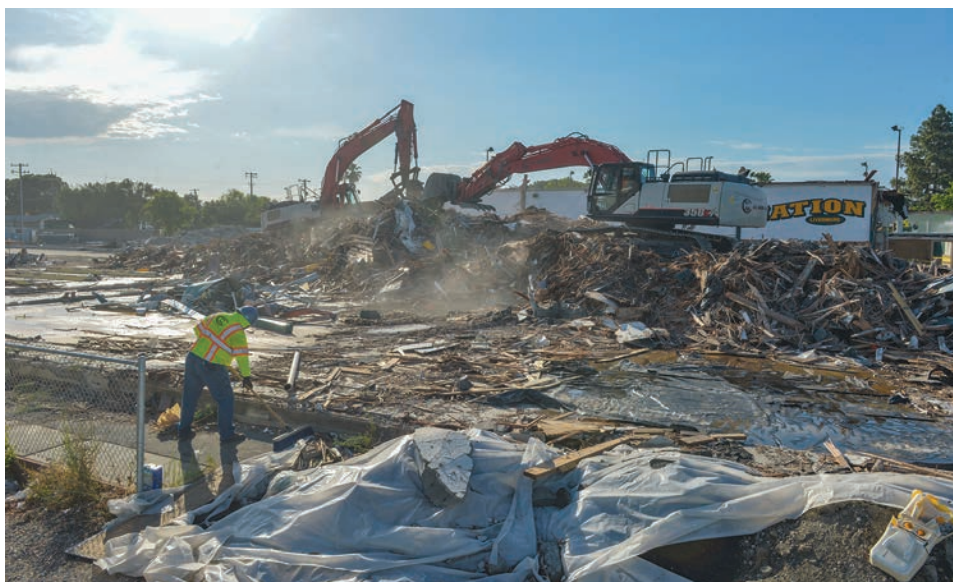
The gymnasium that had served Livermore High School for approximately 65 years, along with the Small Gym, were demolished to begin work on the Livermore High School Aquatic Complex that will include a 12-lane competition pool and water polo field. The Old Gym began as an aircraft hanger at Livermore Naval Air Station (NAS) during World War II. The Livermore NAS was at the site of what is now the Lawrence Livermore National Laboratory. (Photo - Doug Jorgensen)
