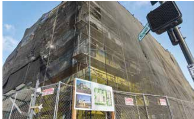
With its general contractor, Katerra, filing for bankruptcy, construction on Legacy Partners’ development in downtown Livermore is on hold. Work will recommence once a new contractor is hired. (Photo – Doug Jorgensen)
