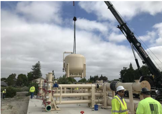
Crews move new treatment vessels to the Zone 7 Water Agency's Stoneridge site in Pleasanton. The new equipment will help bring the site's contaminated wells back into service as early as September. (Photo courtesy of Zone 7 Water)
