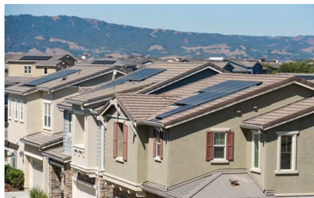
Rooftop solar panels that generate 28.5 gigawatts of power would save 148,000 acres of land needed to develop solar farms, according to a report by Environment California. (Photo – Doug Jorgensen)
