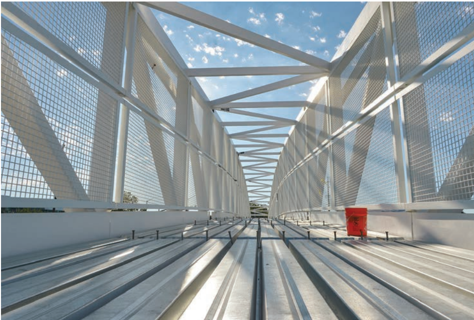
This week’s planned erection of the Iron Horse Trail Bridge overcrossing has been postponed due to unforeseen circumstances, according to the City of Dublin’s website. The bridge is currently sitting on the side of Dublin Boulevard in front of Don Biddle Park. Staff and city consultants are working to determine a new date for the installation. (Photo - Doug Jorgensen)
