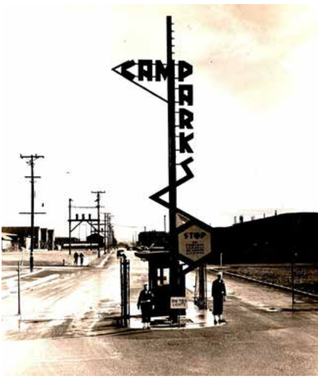
The original Camp Parks gate sign and guard shack, circa 1944, are being restored and relocated to the Dublin Camp Parks Military History Center. The work is expected to be completed by early fall. (Photo courtesy of City of Dublin).
