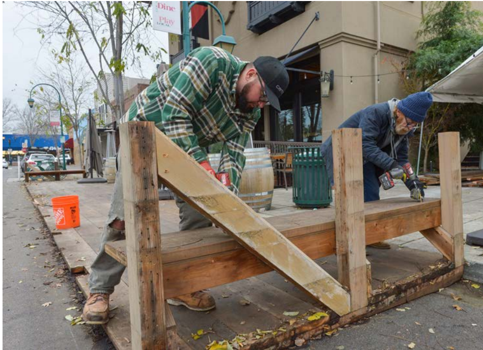
From left, Jake Snyder and Richard Hopper dismantle the parklet in front of Beer Baron on St. Mary’s Street in Pleasanton. The city recently required restaurants and owners to remove the structures, which were originally installed to encourage outdoor dining during the pandemic. (Photo - Doug Jorgensen)
