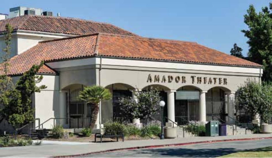
Officials report that the Amador Valley Theater is not closed due to ADA-compliance issues. However, it is in need of major repairs. (Photo – Doug Jorgensen)
