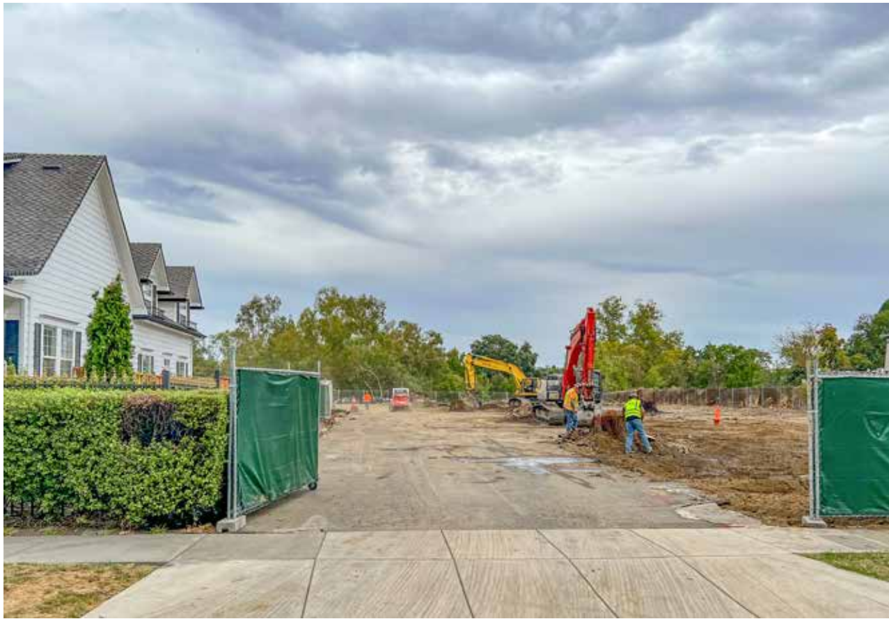
Demolition has begun at the downtown Pleasanton site of the former Barone's Restaurant, a longtime local fixture that closed permanently in October 2024 after nearly 30 years in business. The 2.3-acre parcel has been approved by the City Council for redevelopment, including new homes and a plaza. (Photo — Leah Silveira)
