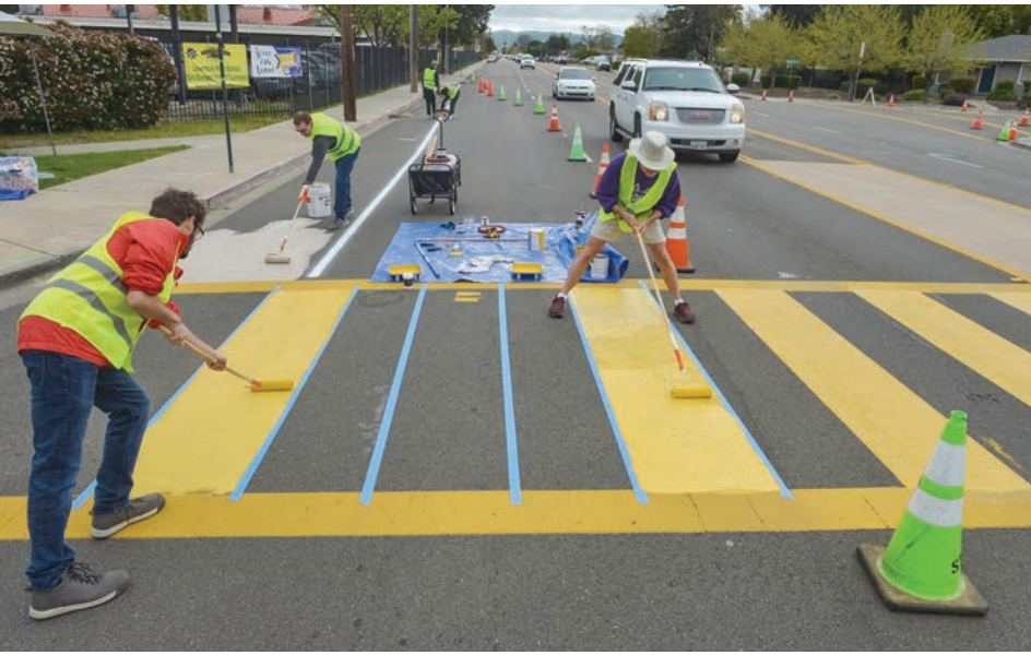
Volunteers Zackary Cosenza and Randy Simpson freshen up the crosswalk at Maple Street and East Avenue in Livermore as part of the Tactical East Avenue, Phase II of the East Avenue Corridor Study. Improvements like curb extensions, pedestrian refuge medians and high visibility crosswalks will be evaluated for six months at the intersections of Maple, Seventh, Dolores, Jensen and Estates streets, as well as Hillcrest Avenue. During the evaluation period, the city will monitor the project, collect data, and solicit public feedback to determine how the project is functioning. (Photo - Doug Jorgensen)
