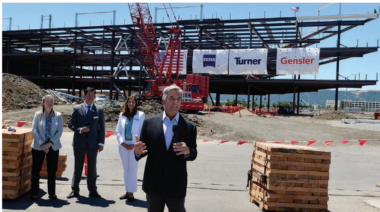
On July 11, a topping out ceremony was held at Carl Zeiss Meditec in Dublin. Topping out refers to placing the last or highest steel beam during construction. The building, located at 5300 Central Pkwy., will serve as the U.S. headquarters for the Zeiss Medical Technology group, the company's Industrial Quality & Research branch, and its Semiconductor Manufacturing Technology division. (Photo – Doug Jorgensen)
