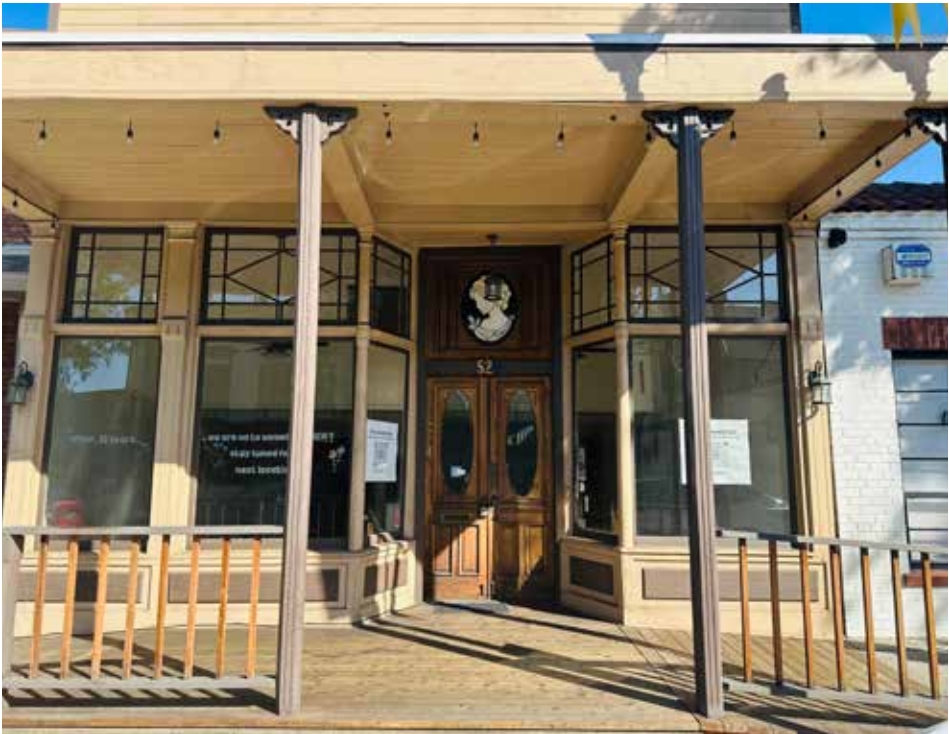
Structural concerns in the building at 520 Main Street in Pleasanton have led to PRIMM Boutique owner Marissa Ringman closing her doors and moving the business to Paso Robles. (Photo — Sanestina Hunter)
