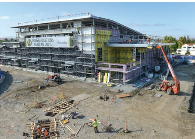
The new athletic and aquatic complex at Livermore High School is on schedule for completion this summer. This project, along with others in the district, was funded by Measure J. (Photo – Doug Jorgensen)
