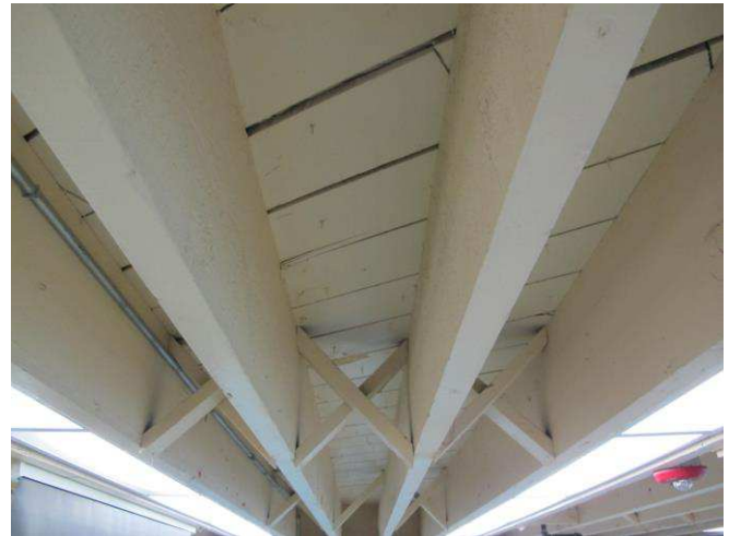
First floor structure of the Dewey Building supported by 2x14 inch joists.
