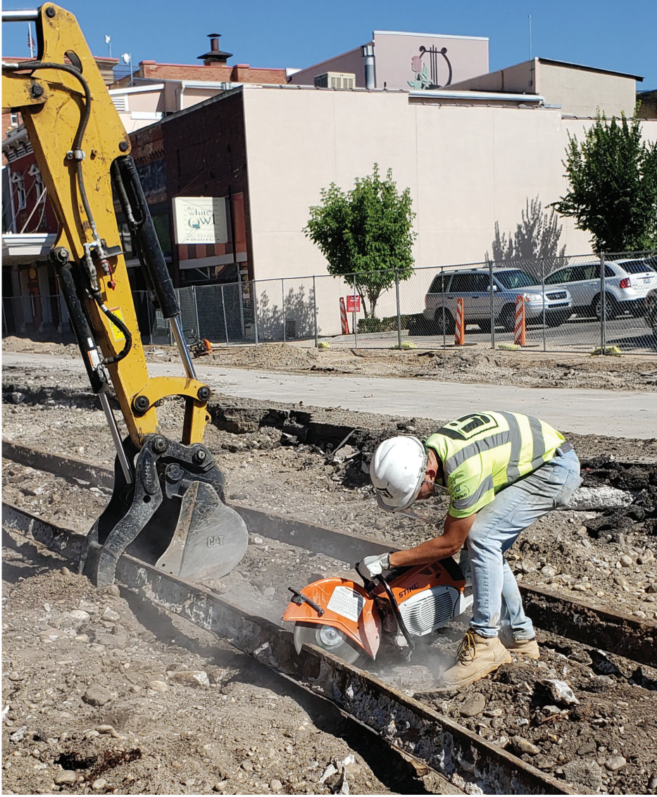
A worker with Legrand Johnson Construction cuts through early 20th century trolley rails unearthed on Center Street in Logan this week.
