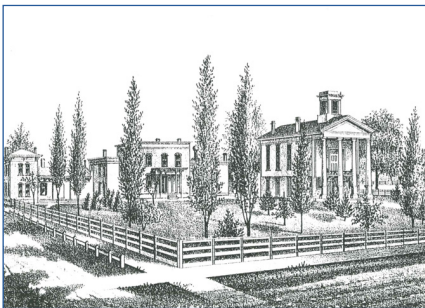
Courthouse, Jail and County buildings - Berrien County Berrien Springs, Michigan 1839
