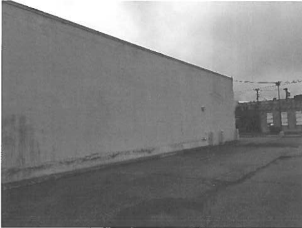
Typical painted masonry veneer (east)
