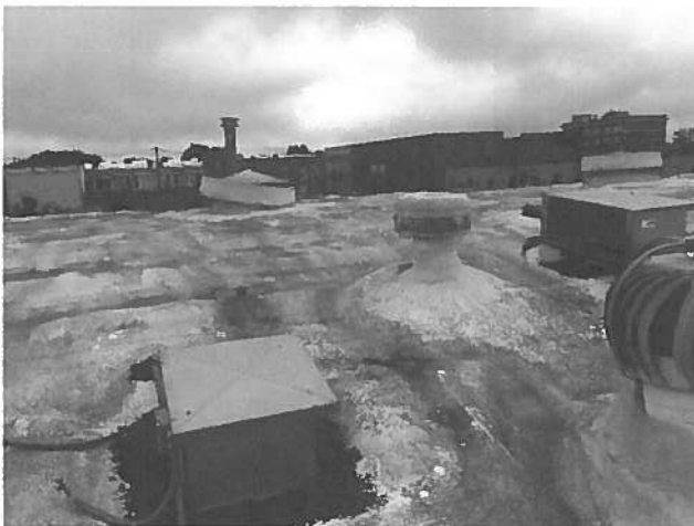
Multiple patches in various roof systems
