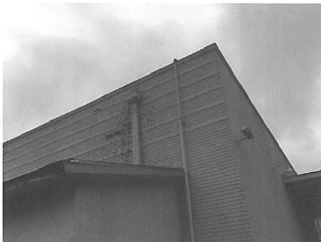
Water issues at lean-to roof and wall in southeast corner of building
