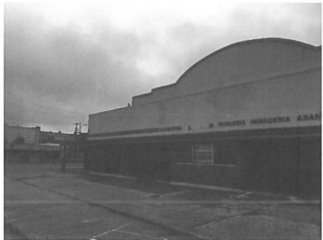
Inadequate handicap accessibility
