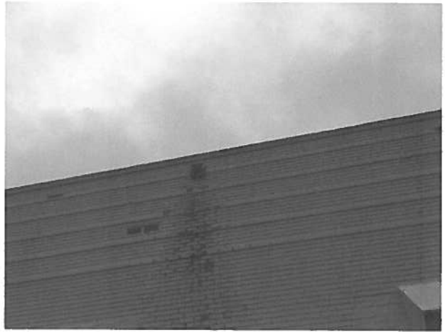
Water runoff through scupper
