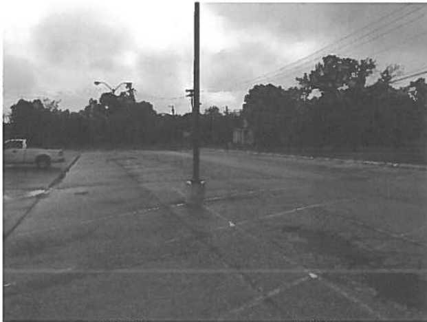
General Condition of the Parking
