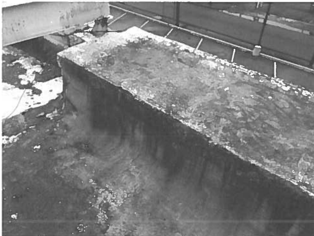
Build up at parapet and cap
