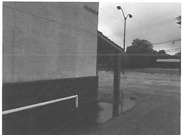
Ponding along north elevation due to lack of positive drainage away from building
