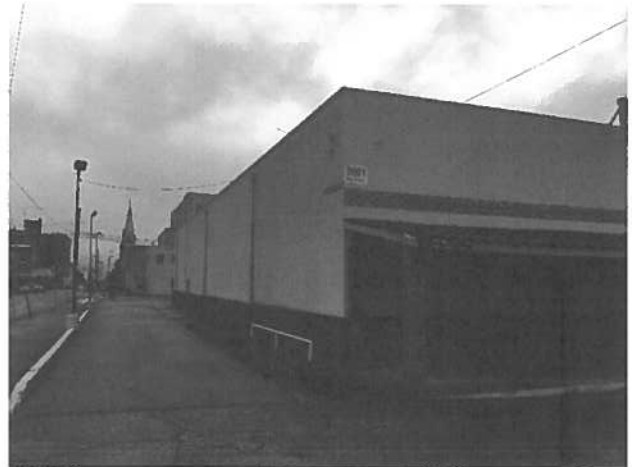
Exposed masonry wainscot (nw)
