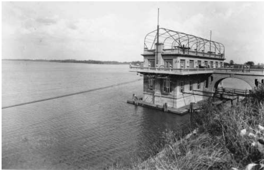
Figure 24. Two early views of the Staley Pump House and Club House. Bottom: Circa 1928 view looking northwest. Top: Undated, pre-1930 view looking northeast ( http://picturedecatour.blogspot.com/2013/12/staley-club-house-pumphouse.html ). Note the low water level and the presence of the floating dock. It appears that by this date a lower level frame bridge had been constructed beneath the Balcony level bridge for accessing the floating docks
