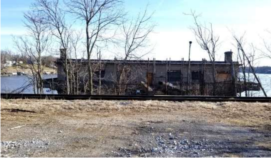
Figure 5, View of the west elevation of the Staley Pump House and Club House from across the railroad causeway.
