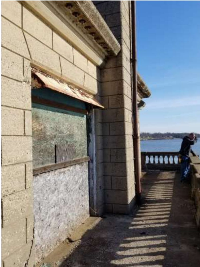
Figure 10. Photographs illustrating the cast concrete, emulating ashlar masonry, and architectural detailing on the Balcony Level of the building. Electric lighting was integrated into the cornice. The photograph at right shows the northern of the two chimneys present on the building.
