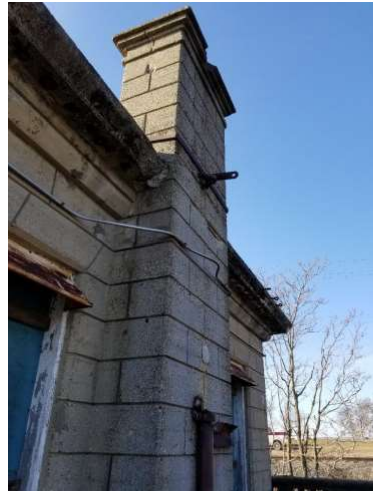
Figure 10. Photographs illustrating the cast concrete, emulating ashlar masonry, and architectural detailing on the Balcony Level of the building. Electric lighting was integrated into the cornice. The photograph at right shows the northern of the two chimneys present on the building.
