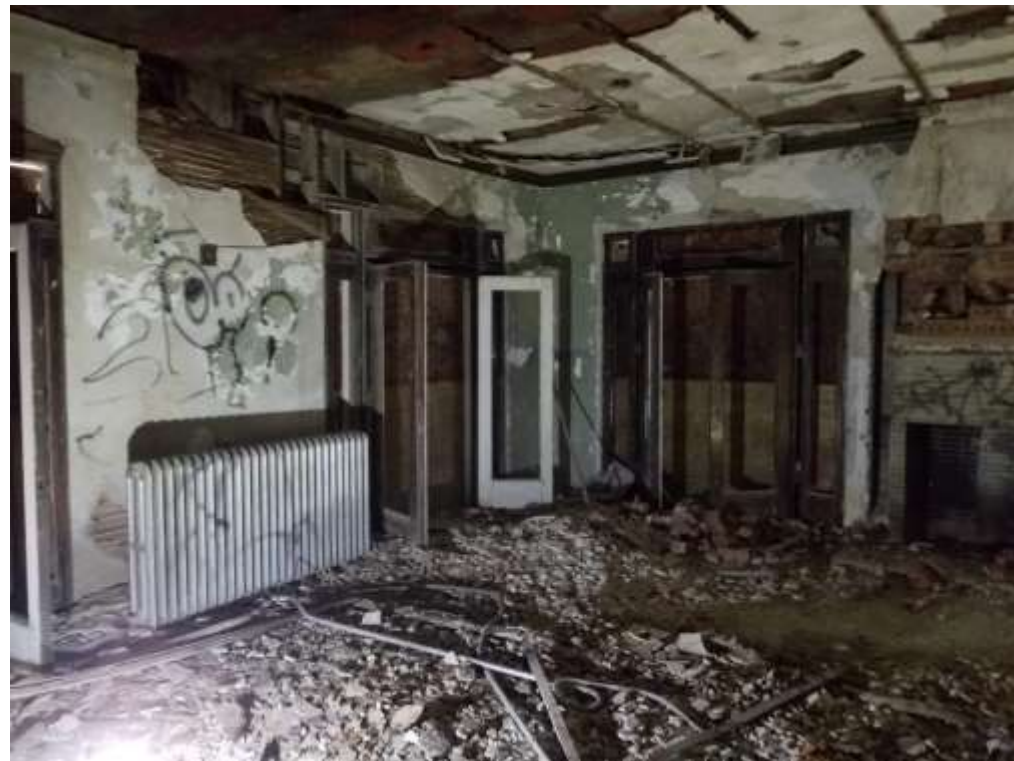
Figure 11. Views of the southern room in the Balcony Level. Note the fireplace and multiple sets of exterior doorways that ring the room. This space originally was used as a dining room.
