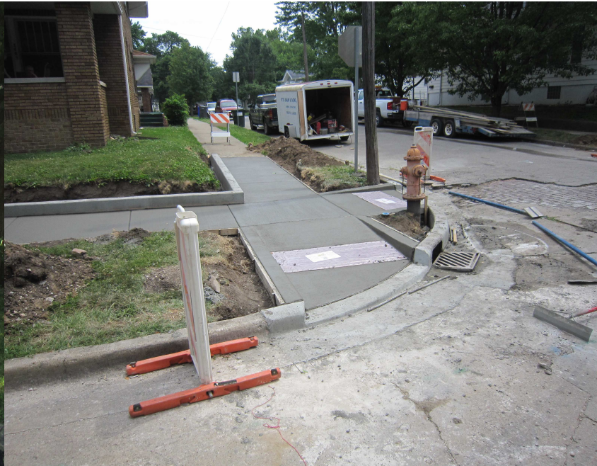
E. Main St. and Stone – New Ramps/curbing
